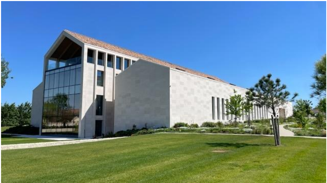
New winery at Leoville Las Cases, opened to the public this year though it has been in use for a couple of vintages.
